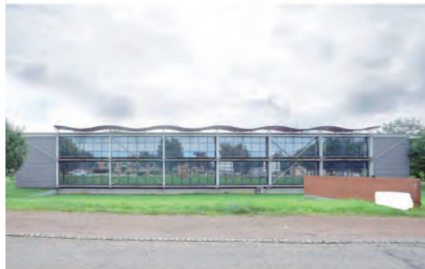
Seriously, did Renzo Piano built here ?
